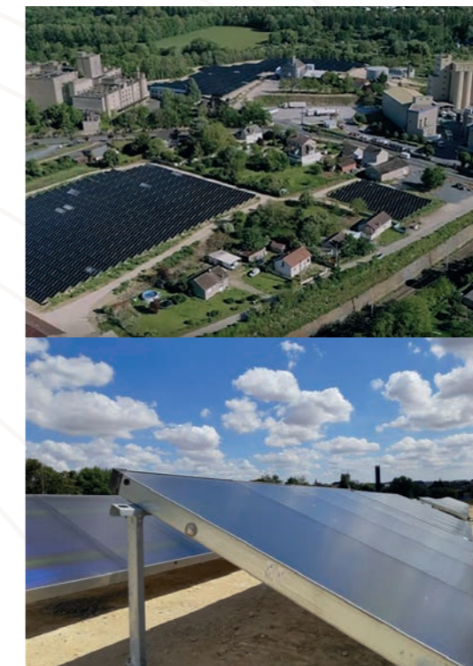
◀ The thermal solar energy plant at our Issoudun malting plant
